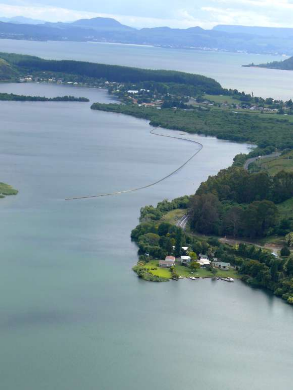
Figure 12. Photo of the Ohau Channel diversion wall, also showing Lake Rotorua (top waterbody). Photo: Environment Bay of Plenty.
