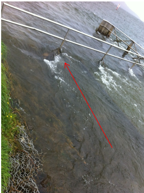
Photo 1. The fish pass can be seen below the log, but appears to be inundated with sediment.
