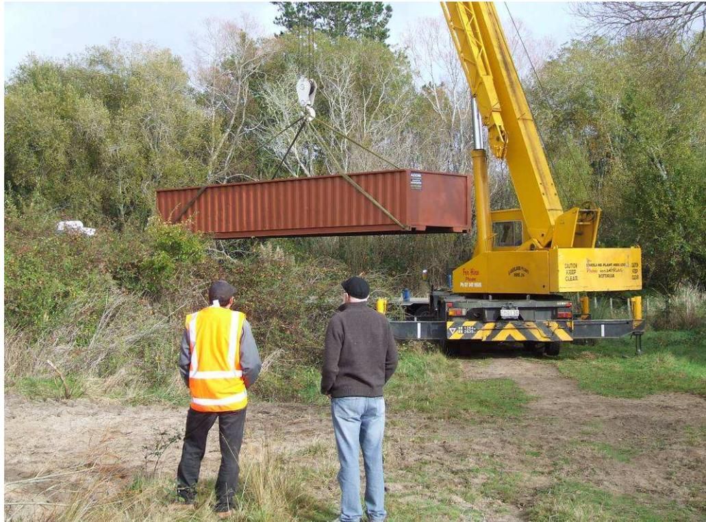
**Figure 4:** Positioning of mesocosm (a modified shipping container) at the experimental site.
