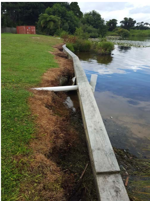
Photograph 25 – Taheke marae retaining wall erosion 160
