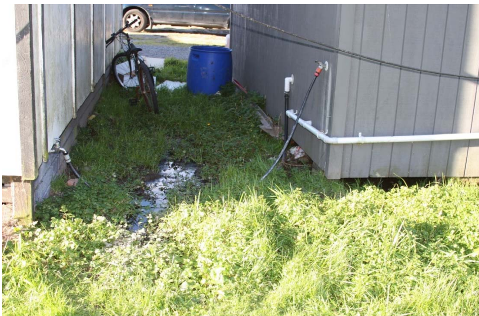
Photograph 35 – Effluent ponding at Ruato Bay 193
