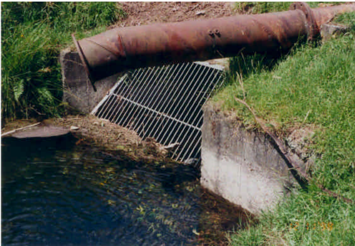
Figure 4 Entrance to pipeline Upper pipe (disused) is remnant of the earlier pump scheme.
