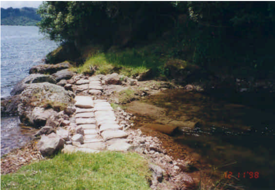
Figure 3 Weir and culverts between lake and outlet canal Not all culverts visible in this photo. Weir has been subsequently rebuilt.
