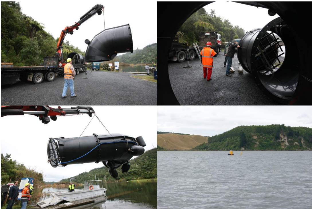
Figure 4. Installation of the mixing devices in Lake Rotoehu. Images by A. Bruere.
