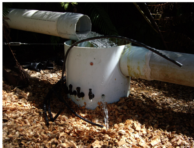
Fig. 1 For reference – headworks March 2007 before top holes were bored.
