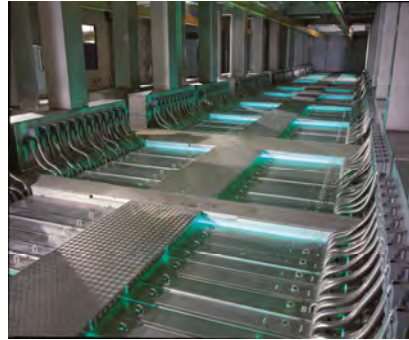
UV disinfection now installed at many NZ wastewater Treatment Plants
