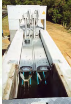
UV disinfection now installed at many NZ wastewater Treatment Plants
