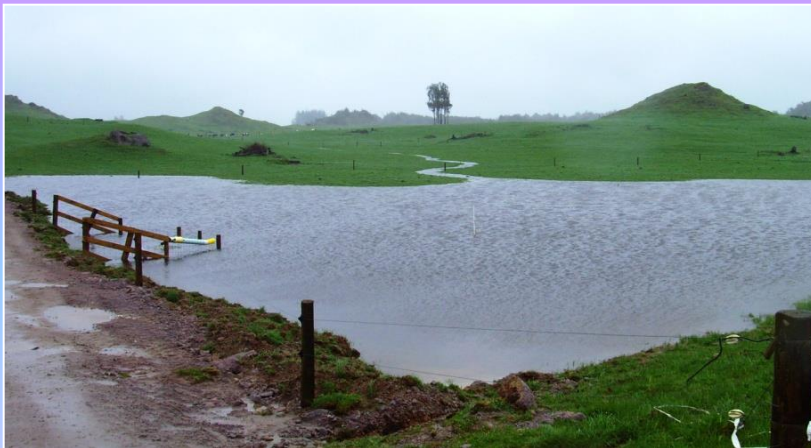
Pilot detainment bund, Rotorua
