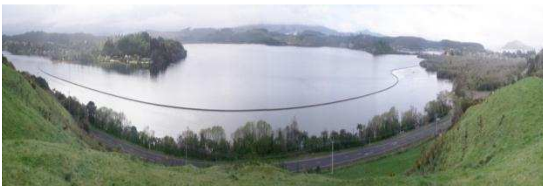
Figure 33. Diversion wall in Lake Rotoiti
