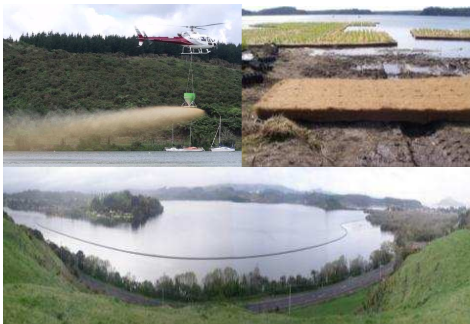
Figure 32. Chemical dosing at Lake Ōkāreka (top left); floating wetland in Lake Rotorua (top right); diversion wall in Lake Rotoiti (bottom)
