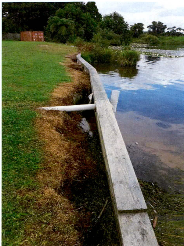
Photograph 25 – Taheke marae retaining wall erosion 160
