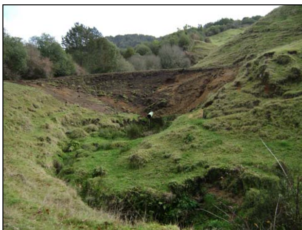
Figure N15.1 Plastic drain pipe with spring flow from soil bank, Paradise Valley Road, looking west.
